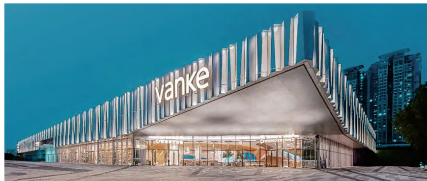
Vanke Huadiwan Life Center in Guangzhou
