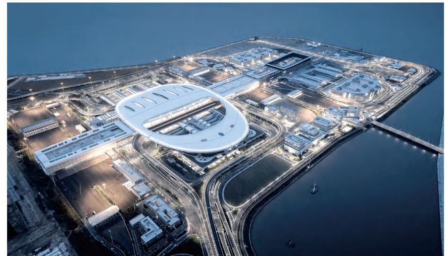
Hong Kong-Zhuhai-Macao Bridge
